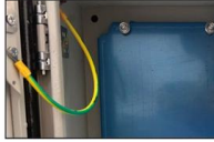
Grounding screw More aesthetically pleasing and safer
