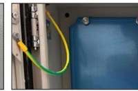
Grounding screw More aesthetically pleasing and safer
