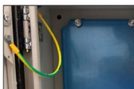
Grounding screw More aesthetically pleasing and safer
